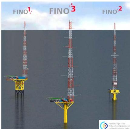
Fig. 1: Mast designs with different foundations. [Source: FuE-Zentrum FH Kiel GmbH].
